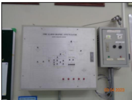
Fire Alarm Graphic Annunciator
